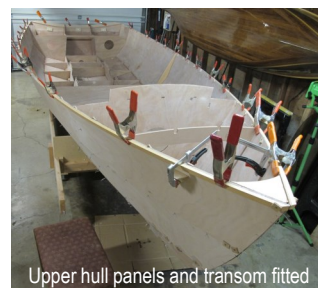
Structural components fitted into hull
