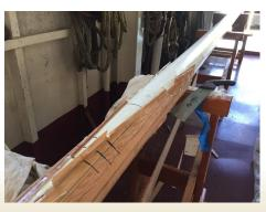
posite sides of the base of the glued upper portion of the mast. The template was used later to cut the matching male portion of the joint on the upper part of the remaining original mast.
